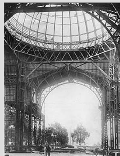
Dome under construction, 1914.
